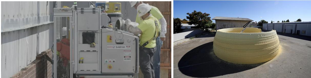
Figure 1.2: (left) Image taken from [4]. A snapshot of Construction Robotics’ SAM100 bricklaying robot at work. (right) Image credit: MIT Media Lab/Steven Keating: A robot that uses visual servoing and the MIT Media Lab’s Print in Place method to 3D print a 14 meter diameter dome out of concrete.
