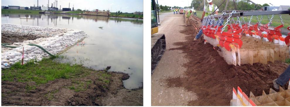
Figure 3.1: From [29]: images of real floodwalls. The structure on the left took 419.8 man-hours to build. The structure on the right requires heavy machinery and human operation in a dangerous flood environment.
